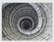
A Large well enables efficient drainage of groundwater in a deep layer.
