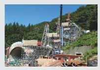
Steel pipe piling is a landslide prevention work of driving steel pipes into the ground to the depth of a few scores of meters. The largest steel pipe piling we have implemented is driving 550 mm-diameter pipes to the depth of 46.5 m.
