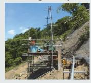
A continuous geological core sample collected in this survey is used to elucidate the geological condition of the site in detail. The drilled borehole is used for measuring underground displacement and groundwater level.
