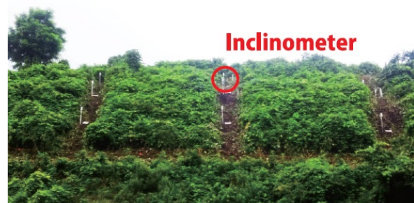
Fig3. Cut slope monitoring
