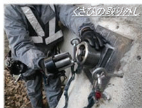
Removal of Wedge
