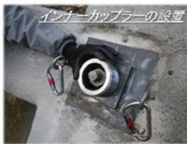
Installation of Inner Coupler
